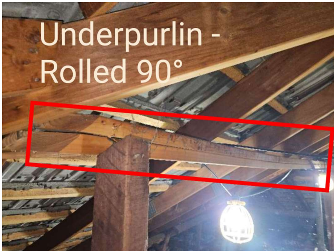
Unevenness/Sagging To Underpurlin From Disproportionate Load
